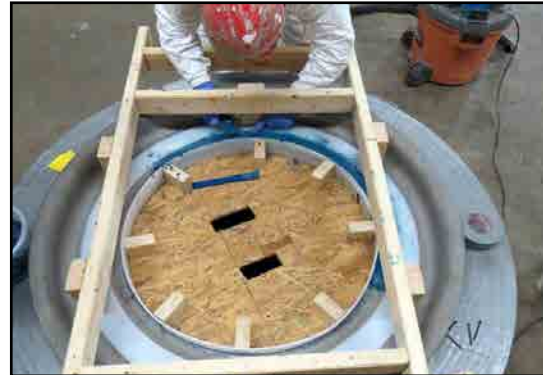
Installing ARC coating to wear region
